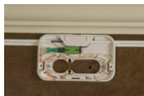
5. Insert connector into adapter.
