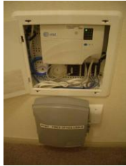
Indoor ONT with mechanical connector
