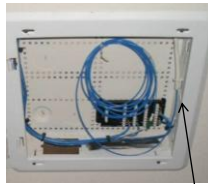
3mm cable pre-installed in microduct
