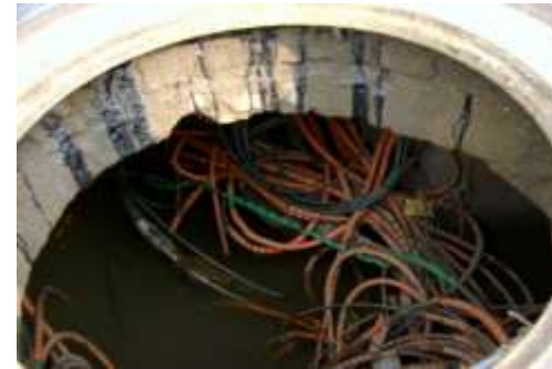
<Outside Plant: Manhole, etc>
